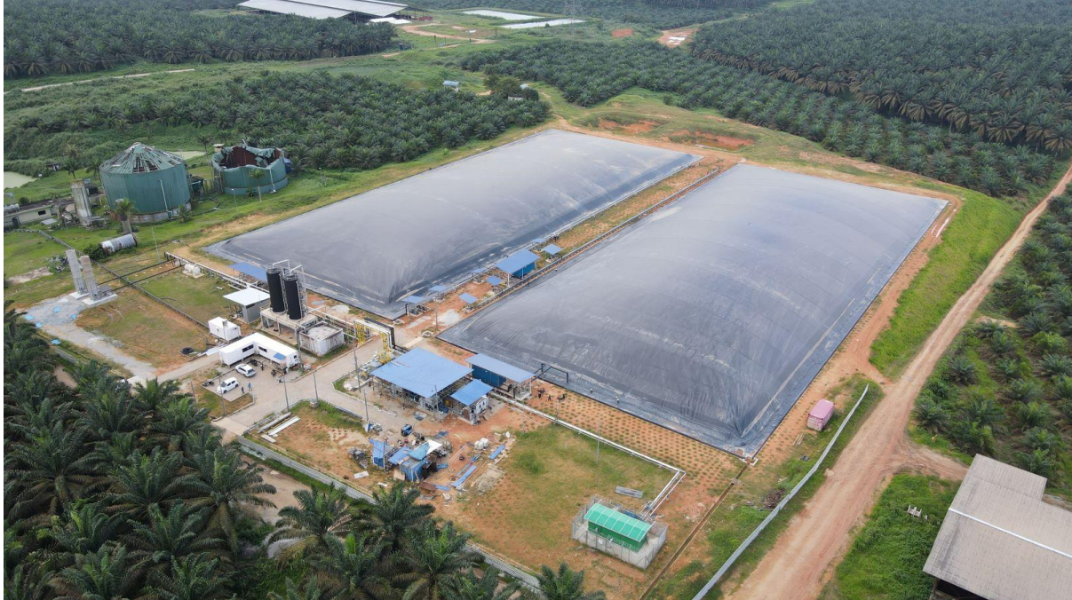
PIC 1: MTC Orec's Biomethane Generation Plant located at Sedenak, Johor.
